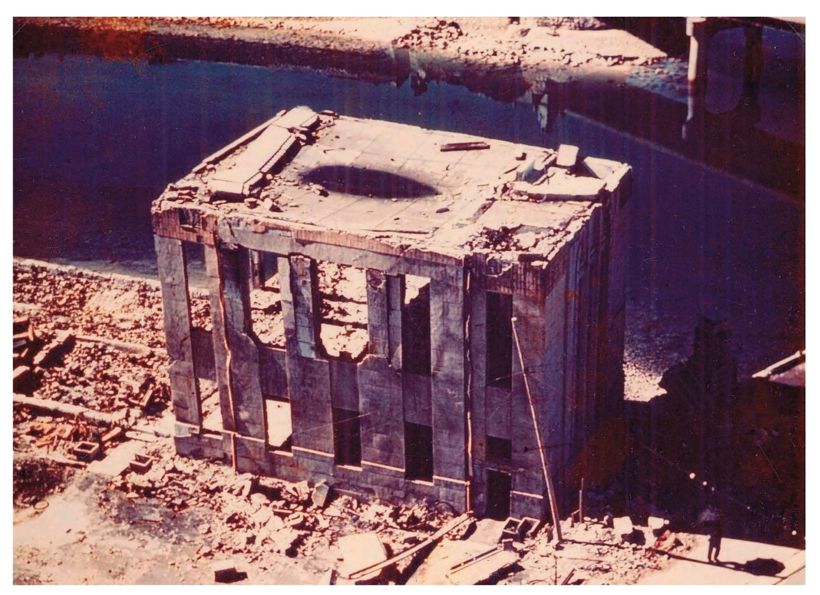
Located directly below the hypocenter, the blast left a large dent on the roof of this building. A typhoon the following September left the large puddle in this dent on the roof as seen in this photo.
