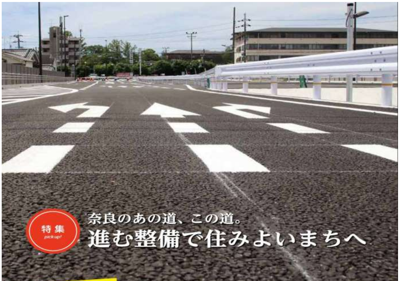
Photo: Shikishima Construction Area of Newly Opened “ Yamato-Chuo-Do Road”
