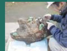
The rocks are reinforced with a chemical substance, then damages and cracks are repaired.
